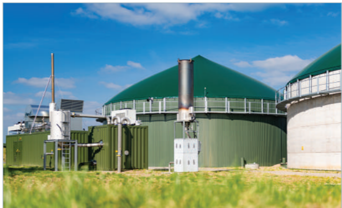
District heating generation
