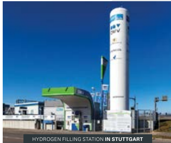
HYDROGEN FILLING STATION IN STUTTART
